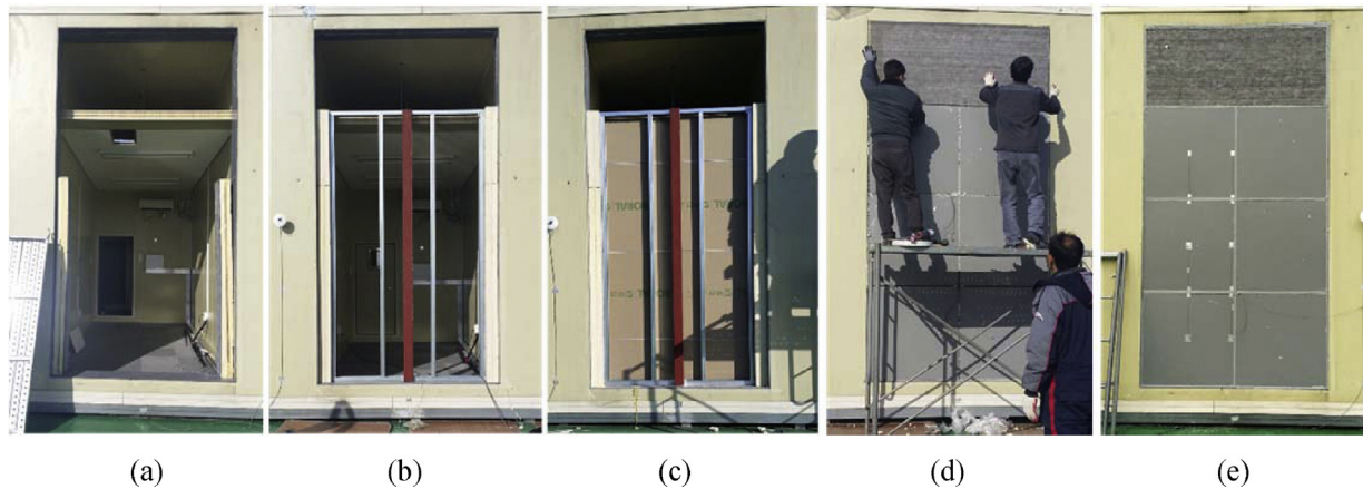
Fig. 14. Installation of specimen: (a) Urethane boards, (b) Vertical truss for fixing metal panels and steel frame for fixing gypsum boards, (c) Gypsum boards, (d) Metal panels and urethane boards, and (e) Joint sealing and sensors.
